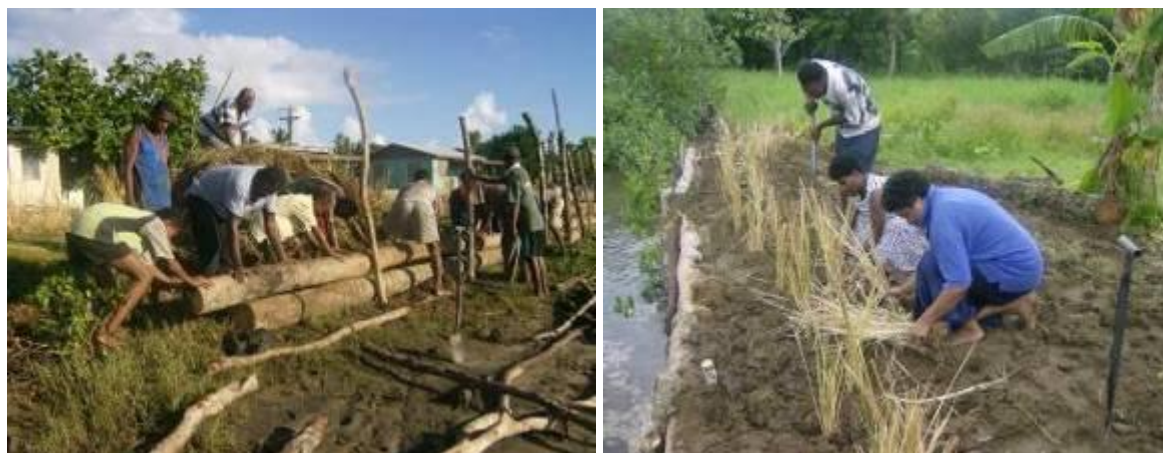
Construction of river bank protection structures using local materials, and planting of vetiver grass for bank stabilization (Buretu, Fiji – USP CBA project)
